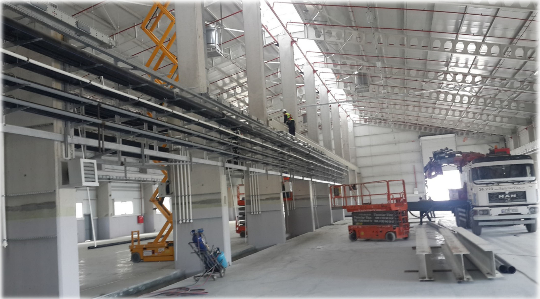
Mutlu Battery, Steel Construction, Crane and Process Piping System
